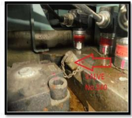
Sampling Valves are installed at a point in the system where the flow is normally constant and turbulent. To obtain representative sample, it is essential that only new and clean samples bottles are used. Valve number 340 is a suitable oil sampling point.
